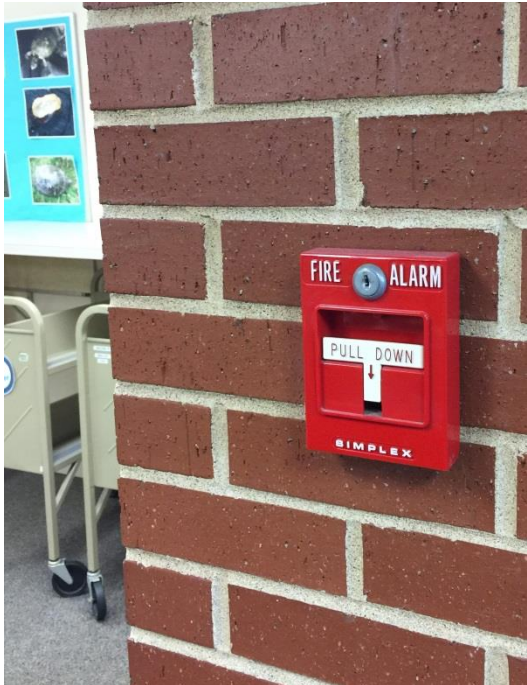
A Typical Pull Station:
